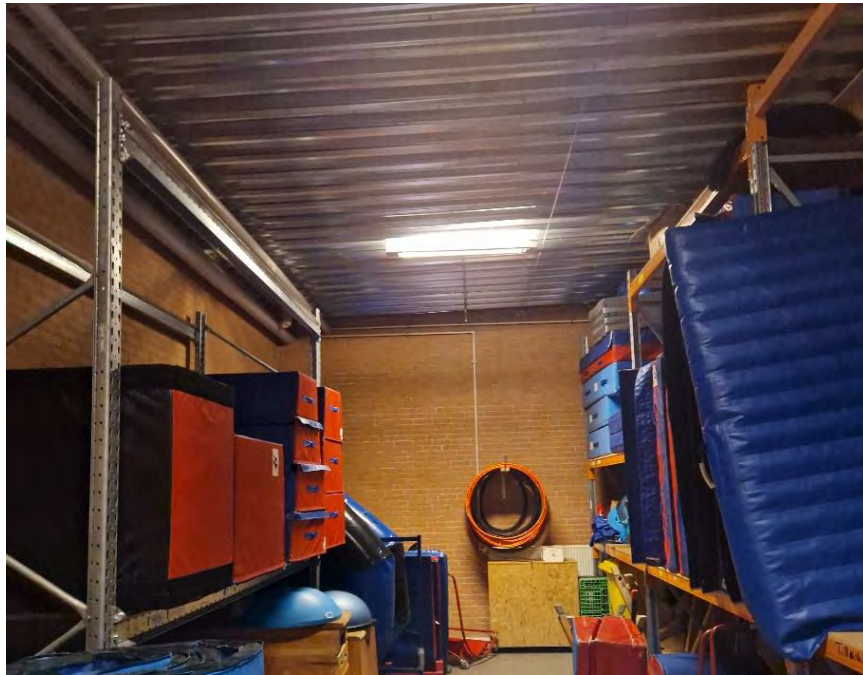
Figur 80: Stål trapezloft i depot.
